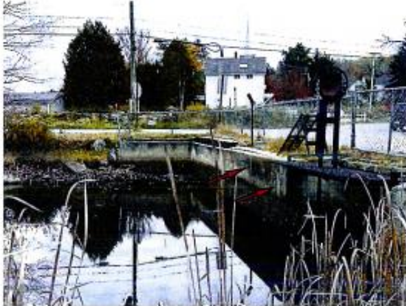
A - Upstream Left Side
